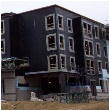
*Liquid applied air barrier installation with sheet applied transition membranes at openings. Photo courtesy of Len Anastasi*
