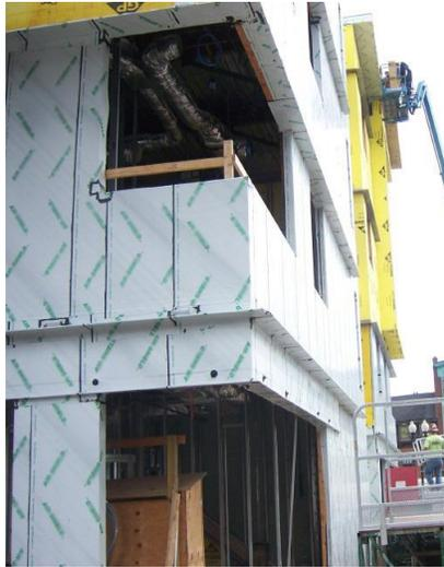
*Air barrier installation around openings and projections. Photo courtesy of Len Anastasi*
